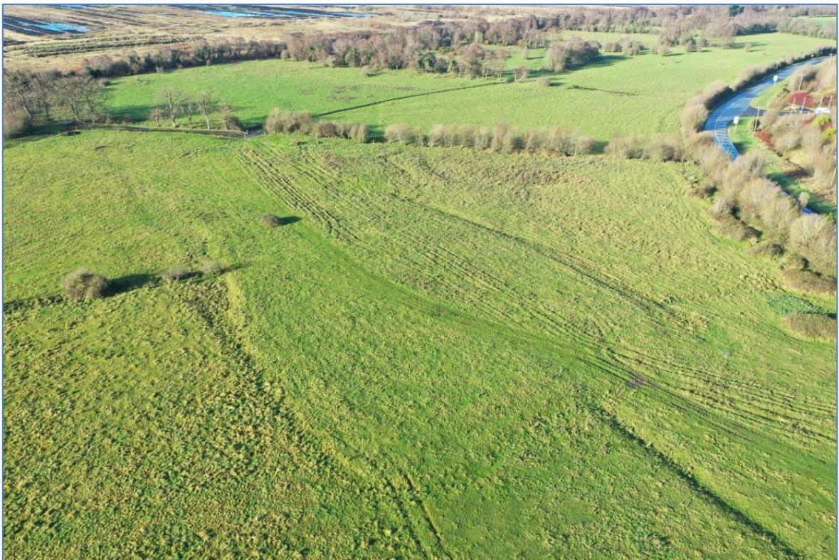
Plate 10-5: Oblique low flown aerial image from SE of the proposed Kilcumber Bridge 110kV substation site (LDARCH).
