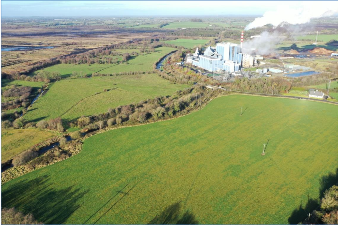
Plate 10-6: Oblique low flown aerial image from S of the proposed Kilcumber Bridge 110kV substation site opposite Edenderry Power Plant (LDARCH).
